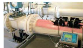
Clamp-on sensors are quickly installed, without interrupting gas flow.
