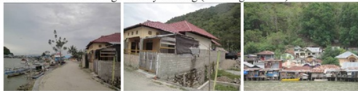
Fig. 12: Uncontrolled construction in riverside area.
