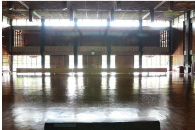
Figure 6: The interior of Salman Mosque, it's free of column, one of the Noe'man design character. Private Collection, 2012
