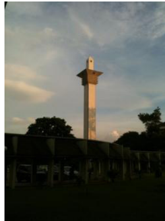
Figure 24: Still the same tower. Aditya, Nova Chandra Collection 2011.
