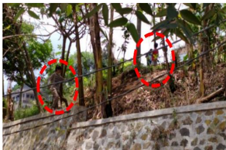
Figure 13. “Dangerous” Access Spaces
