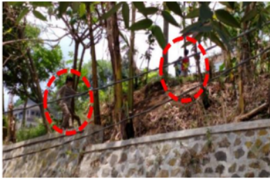
Figure 13. "Dangerous" Access Spaces
