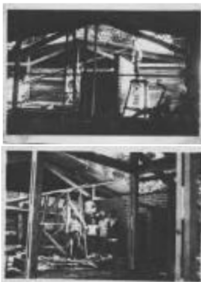
Figure 5. Mushala prior to the construction of the Salman Mosque
