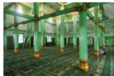
Figure 26. Ornaments on the column of Masjid Giri Mosque, showing tripartite division: head, body and foot. Green colour scheme which gives a sense of tranquility is widely adopted in mosques in Indonesia. Source: http://1.bp.blogspot.com , retrieved January 20 2012
