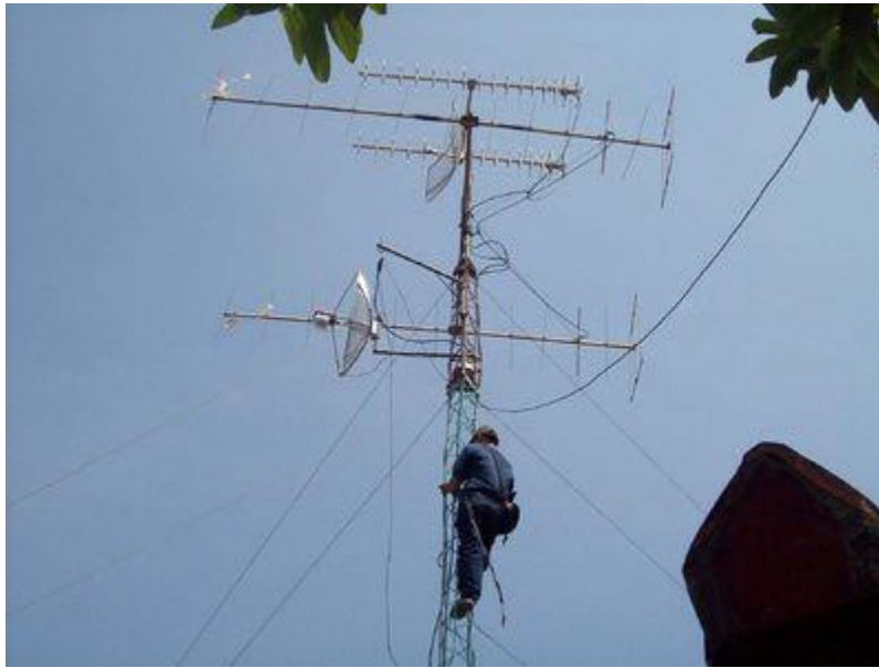
Pemasangan Antena Hand Made 2.4 Ghz
