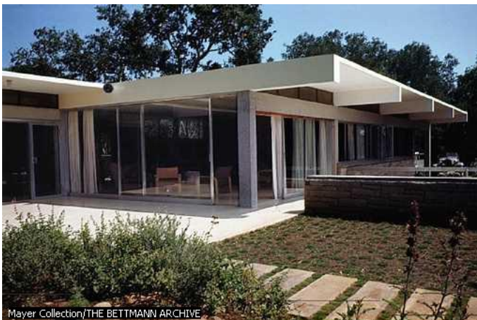
Tremaine House, Santa Barbara Similar in style to Lovell House, his best-known building, the Tremaine House (1947-1948) is an excellent example of the distinctive International Style of Austrian American architect Richard Neutra. The clean lines produced by the combination of concrete and large windows give the home an elegant simplicity, while the overhanging roof and patio create a link between the building and its natural surroundings. Mayer Collection/THE BETTMANN ARCHIVE. Microsoft © Encarta © 2009. © 1993-2008 Microsoft Corporation. All rights reserved.
