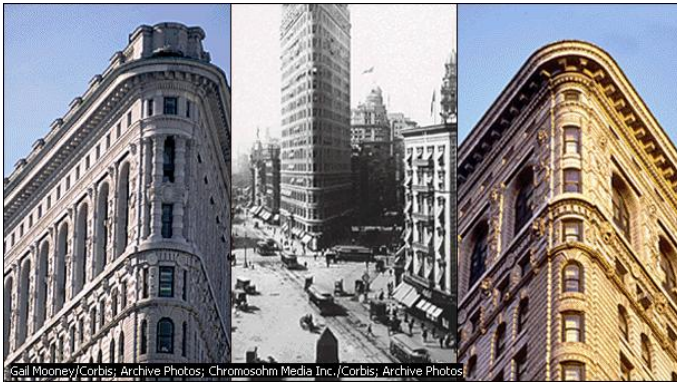
Three Views of the Flatiron Building Completed in 1902, the Flatiron Building in New York City was once the city's tallest building at 91 m (300 ft) tall. Designed by Chicago School architect Daniel Burnham, the triangular building features a decorative exterior supported by a steel skeleton. The Chicago School was composed of architects from Chicago, Illinois, who built some of the first skyscrapers in the United States. Gail Mooney/Corbis; Archive Photos; Chromosohm Media Inc./Corbis; Archive Photos. Microsoft © Encarta © 2009. © 1993-2008 Microsoft Corporation. All rights reserved.
