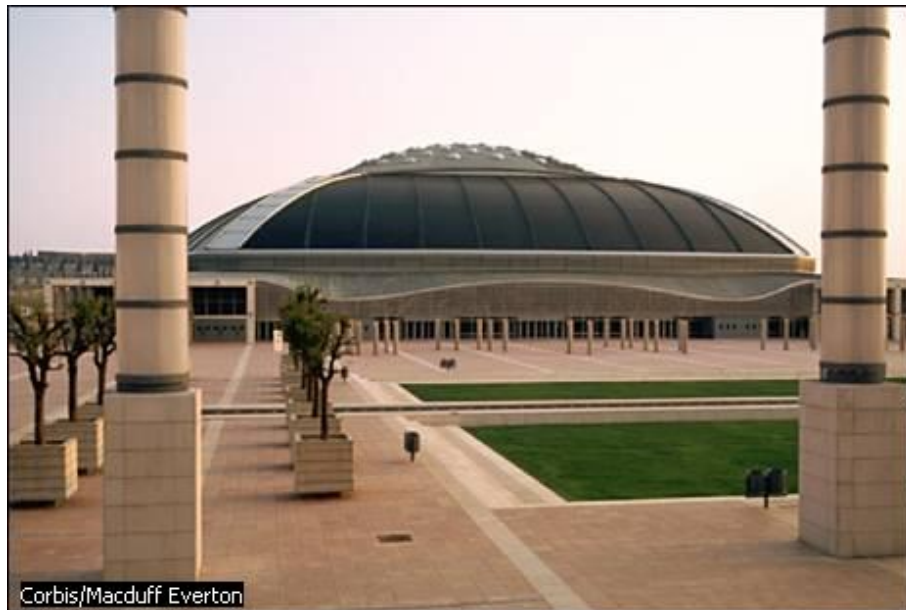
Palau Sant Jordi Sports Pavilion. Japanese architect Arata Isozaki designed the Palau Sant Jordi Sports Pavilion in Barcelona, Spain, for the 1992 Summer Olympic Games. Isozaki's designs are renowned for their blending of Eastern and Western architecture styles and their graceful, curved lines. Isozaki also designed the Museum of Contemporary Art in Los Angeles. Corbis/Macduff Everton. Microsoft ® Encarta ® 2006. © 1993-2005 Microsoft Corporation. All rights reserved.
