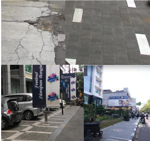
Gambar 5. Warna material trotoar.
