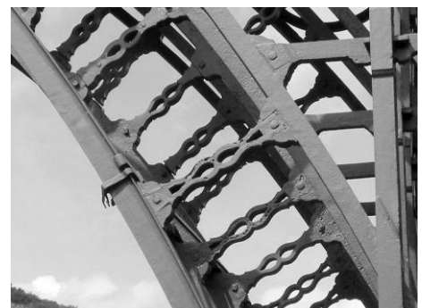
Being the first bridge to be made from cast iron, there was no precedent for the design. A lot of woodworking techniques were used, because that was what you used in those days for building bridges. So, you get things like this - a cast iron dovetail joint.
