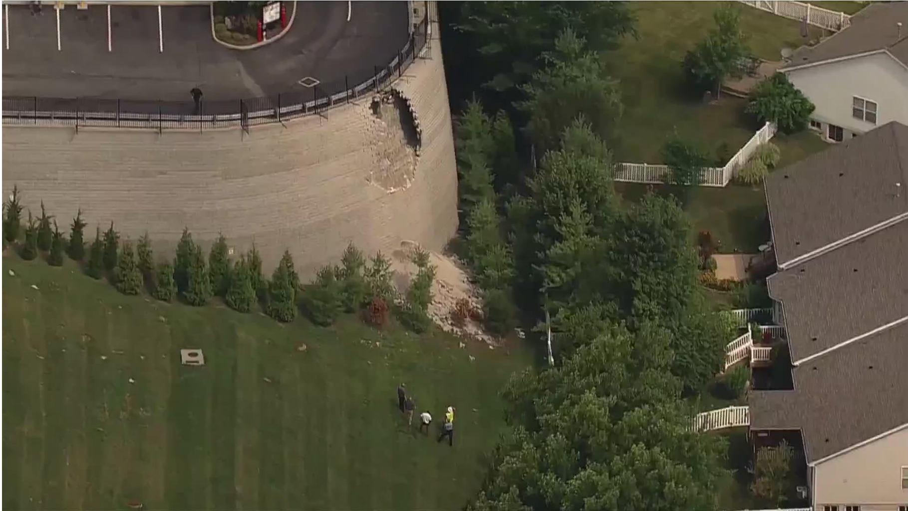
Collapsed retaining wall in Arnold drew concerns over cracking five years ago
